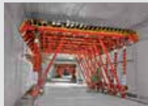
Tunnel Formwork
