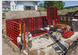
Wall Formwork
