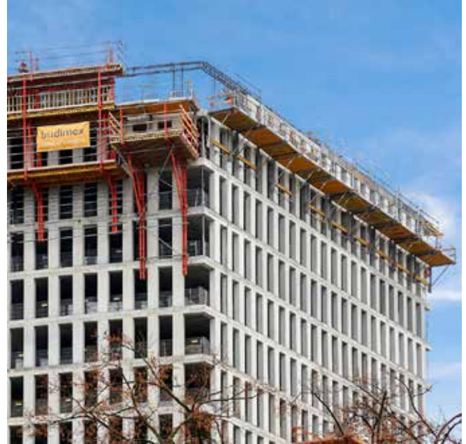
On-site assembly of the Folding Platform FB 180 proved to be quick and straightforward as it was delivered to the construction site in a pre-assembled state.
