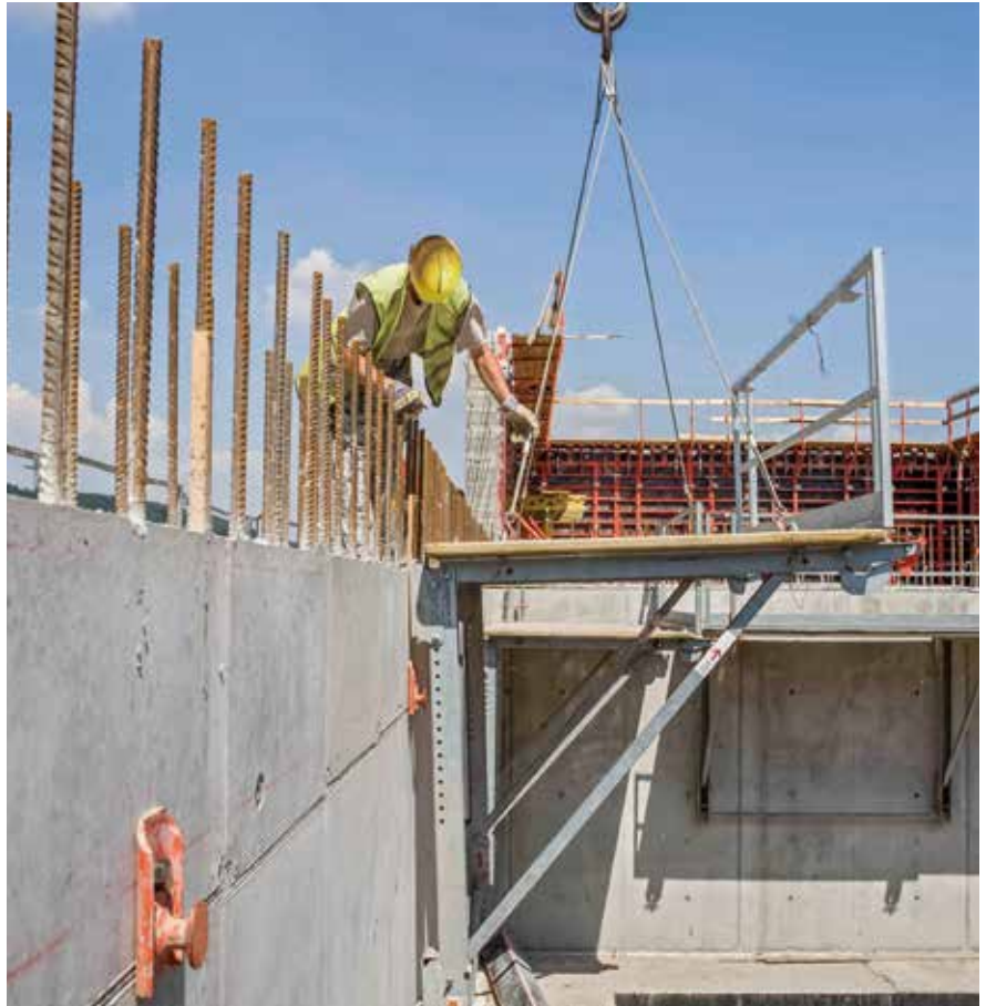
The folding platform is mounted on site and can be quickly lifted into position using four-sling lifting gear.
