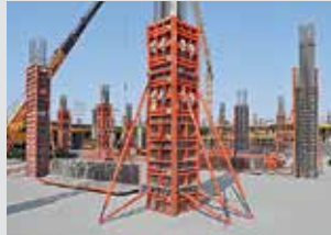
Column Formwork
