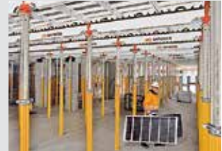
Slab Formwork
