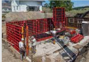
Wall Formwork
