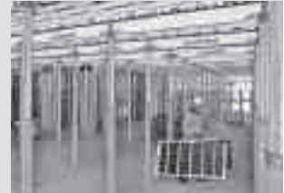
Slab Formwork
