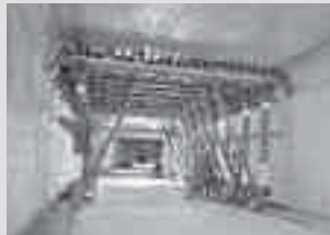
Tunnel Formwork
