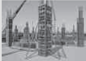
Column Formwork
