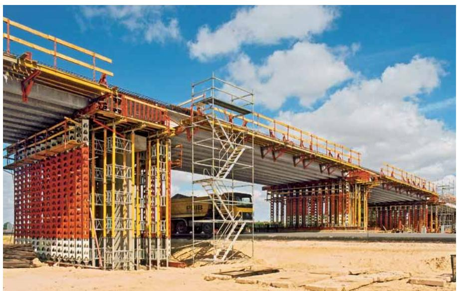
For the construction of this bridge, HD 200 main beam areas were used directly to support the precast girders of the superstructure.
