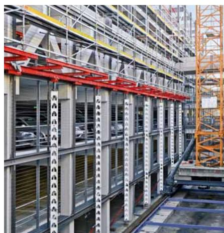
HD 200 heavy-duty props as a space-saving solution: 8 m high props transfer the loads from a working and safety scaffold in a confined area.
