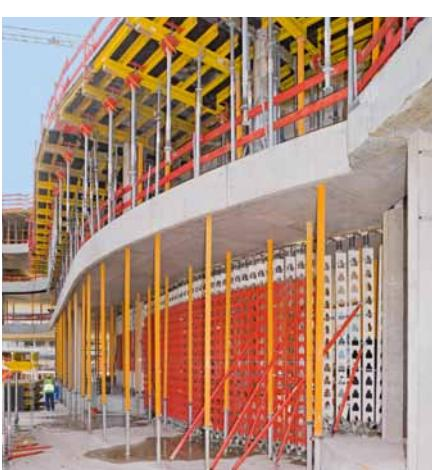
A lightweight but load-bearing solution: Below the shear walls, HD 200 heavy-duty props transfer linear loads of up to 400 kN/m into the bottom plate.
