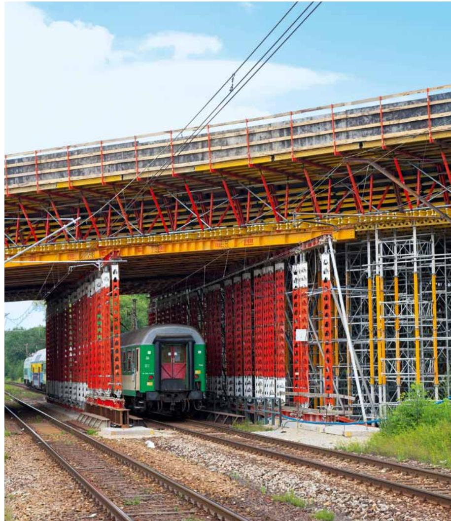
With this portal-like shoring construction comprised of standard components taken from the HD 200 heavy-duty system, traffic could flow freely during the construction period. In the
