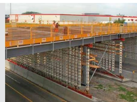
HD 200 as a main beam section for the building of a road crossing using a steel composite construction method.
