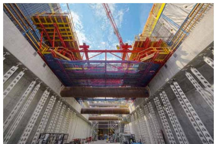
For this underground structure, HD 200 individual props reliably carry the high loads resulting from the subsequent construction work.
