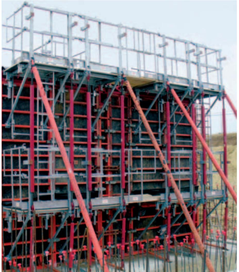
The high rigidity of the panels and the panel connection allow concreting at large heights. As a result, the MXP platform provides maximum working safety.
