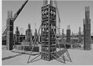
Column Formwork
