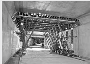
Tunnel Formwork
