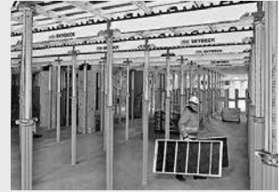
Slab Formwork
