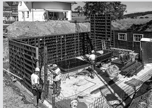
Wall formwork
