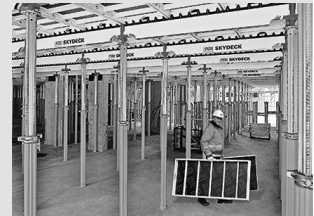
Slab formwork
