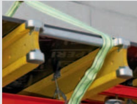
The securely-mounted edge protector provides reliable protection against damage to the formlining.
