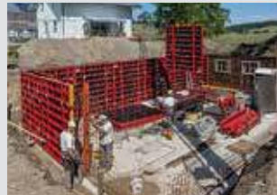
Wall Formwork
