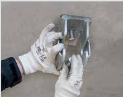
Step 4 Mounting the the Suspension Head VGK with nut M24
