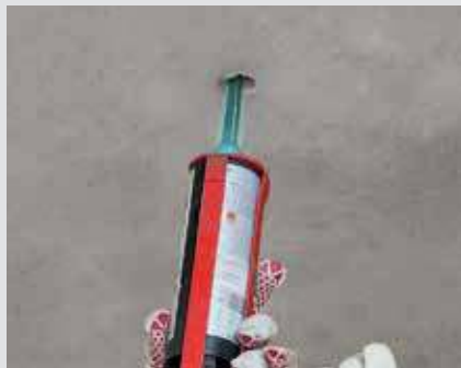
Step 2 Injecting the composite mortar
