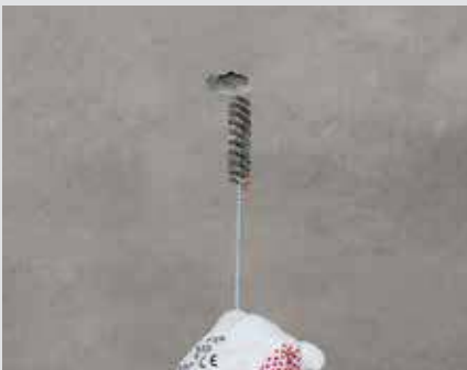
Step 1 Drill hole with d = 22 \text{ mm} and t = 160 \text{ mm} (at right angles to the concrete surface); cleaning the drilled hole with brush and blow-out pump
