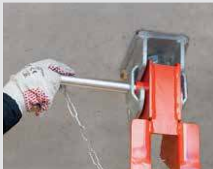
Step 5 Fixing the VGK with bolts
