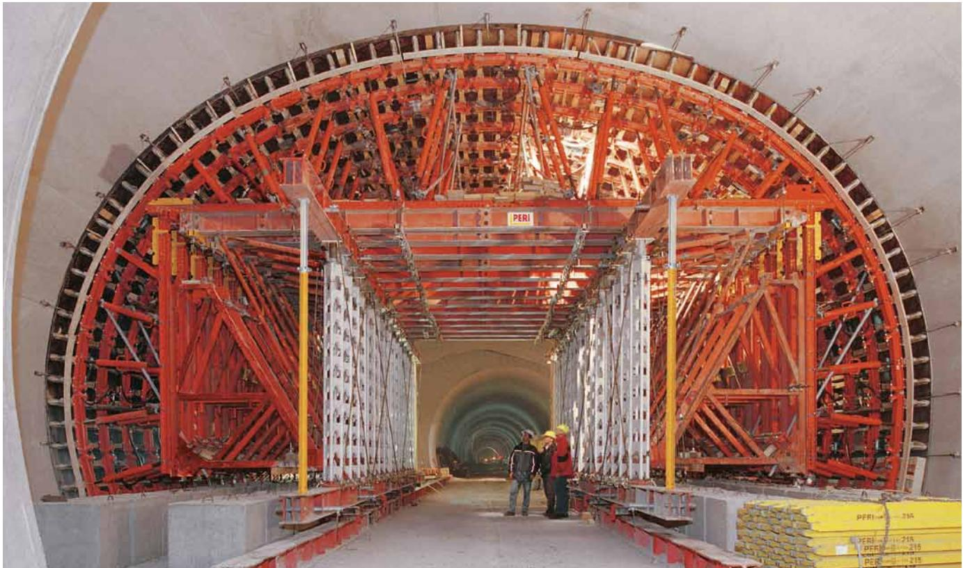
The moveable longitudinal truss - taken from the HD 200 heavy-duty system - for this tunnel was designed as a portal. This allowed a continuous flow of site traffic at all times.
