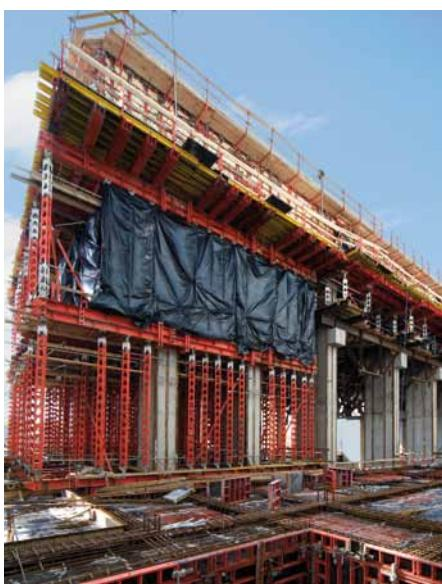
HD 200 heavy-duty props as a full-surface shoring structure. The HD 200 sections were joined together, also at great heights, in order to safely transfer the loads of the 3.20 m thick reinforced concrete slab for the generator.
