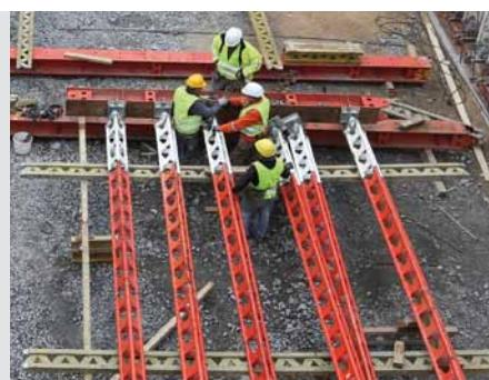
The main beam area is normally assembled horizontally - complete with diagonal bracing, working platform and access ladder.
