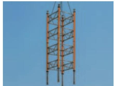
The complete tower can be erected and moved as a complete unit with one crane lift.
