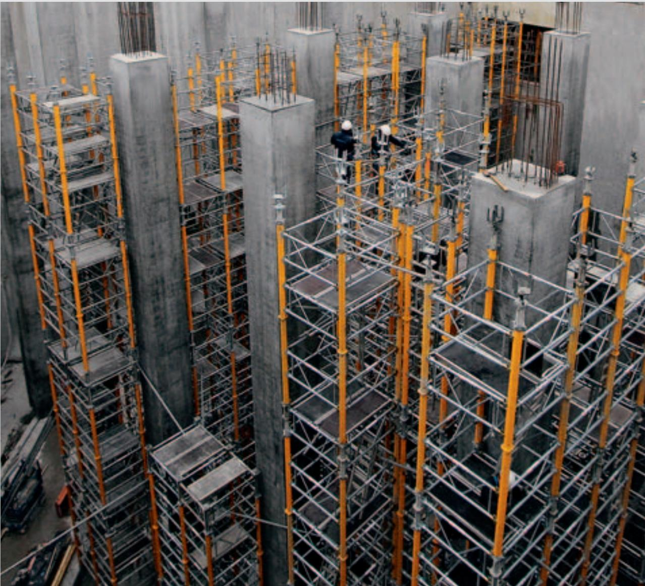
Decking with lengths of 150 cm and 225 cm – with and without access hatches for ladders respectively – allow the installation of shoring with assembly levels and access by means of telescopic ladders.
