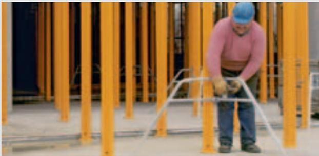
The Universal Tripod serves as a fast assembly aid and accommodates all props from Ø 48 mm to 120 mm.
