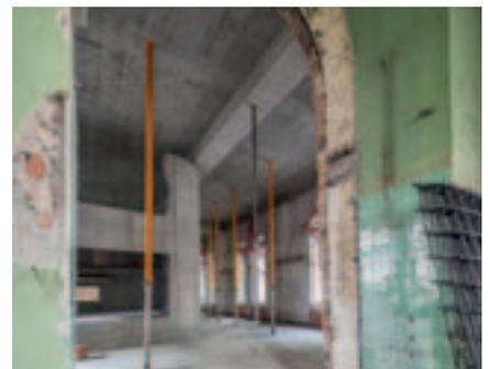
Particularly during refurbishment projects or modification work, MULTIPROP Slab Props allow working without a crane. They are easily transported and positioned by hand.
