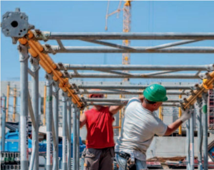
**For the erection of a shoring tower MULTIPROP Frames are connected to the MULTIPROP Props by means of the captive Wedge Coupler. The attachment of the MRK Frame is possible on both the outer as well as inner tube without having any effect on the ground plan.**
