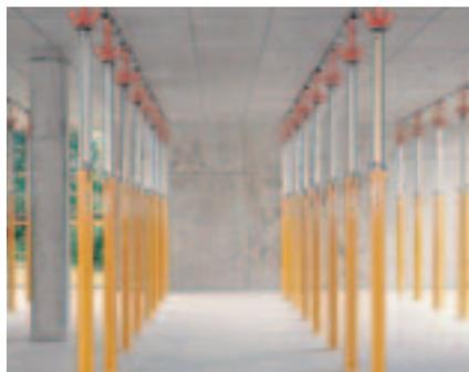
When used with SKYDECK Slab Formwork – shown here after a successful early striking – only 1 MULTIPROP Prop per 3.45 m<sup>2</sup> of slab area is required for a slab thickness up to 43 cm.
