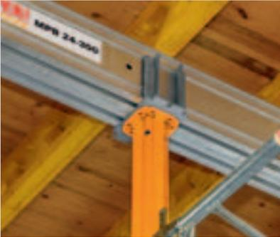
MULTIPROP towers with aluminium MPB Beams as main beams and GT 24 as decking support. Tilting Forkheads provide secure, non-tilting support for the beams.
