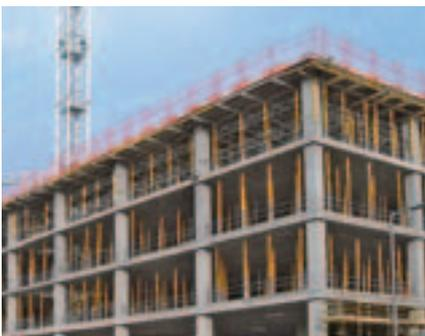
As an individual prop, the MULTIPROP post shore braced with the MULTIPROP Frames MRK carries a load of up to 100 kN per leg. Thus, MULTIPROP is also ideal for the re-shoring of slabs.
