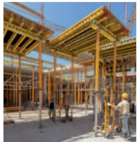
For moving tables or towers, two transportation trolleys are positioned centrally on the narrow frame sides of the shoring, and lifted uniformly.
